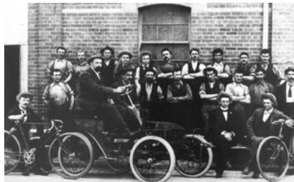
Image above: Adelaide's first petrol-driven car, the original Lewis, pictured on its completion in November 1900. Vivian Lewis is at the wheel and Tom O'Grady is beside him. Murray Aunger, who helped in its construction is seated immediately to the right of the front wheels. Image source: State Library of South Australia
